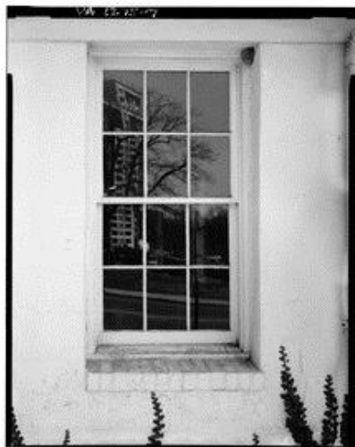
Sash windows are made of one or more panels, or sashes, that form a frame to hold panes of glass. (Wikipedia)
